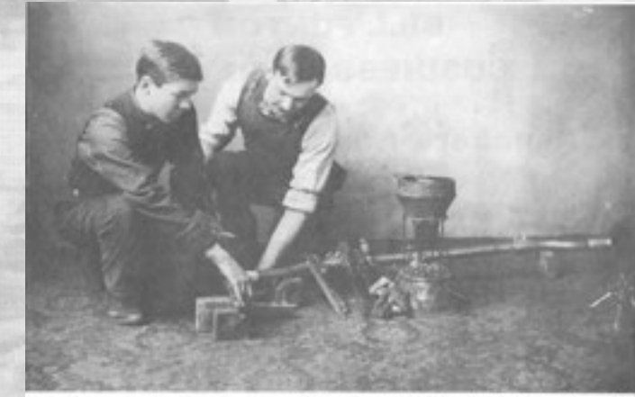
This photograph, taken back in 1908 and submitted by Jim Giffel, shows 17 year old Louis Giffel (left) a Plumber Apprentice and Journeyman Plumber Albert Barna (right). The men were employed at the Fred Arleth Plumbing Shop located at 1315 E. Main Street in Terre Haute.
