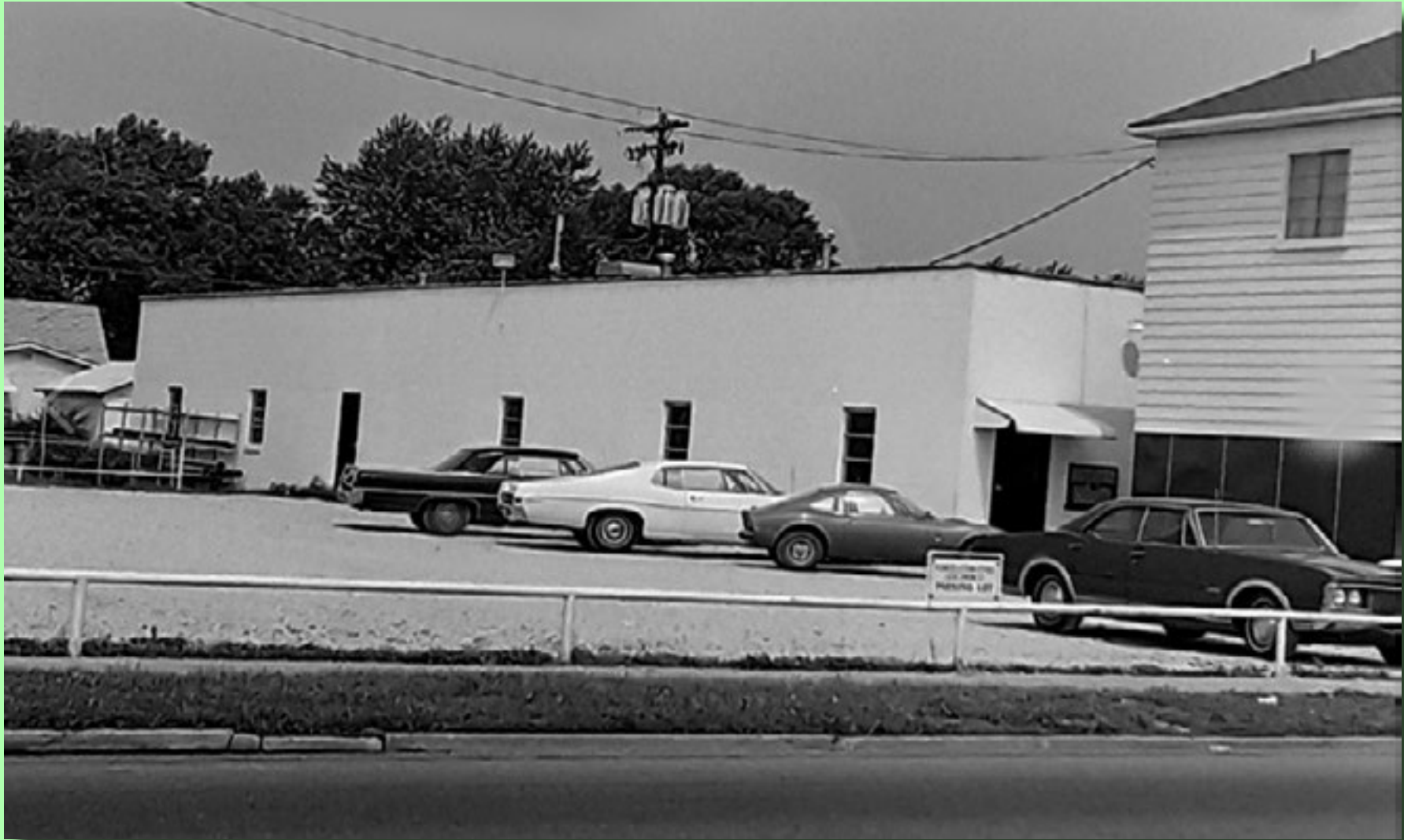
Apprentice Training Building behind 157 Union Hall N. 13th Street.
