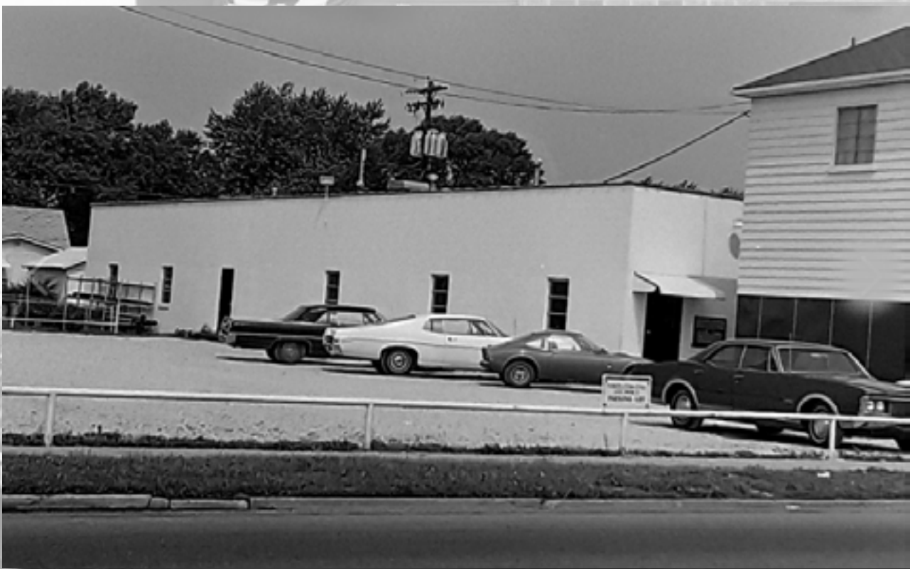
The construction of the Apprentice Building behind the Union Hall on 13th Street allowed the Local's members (for the first time) to train at their own facilities. Up to that point they had been holding classes at Gerstmeyer Technical High School.
