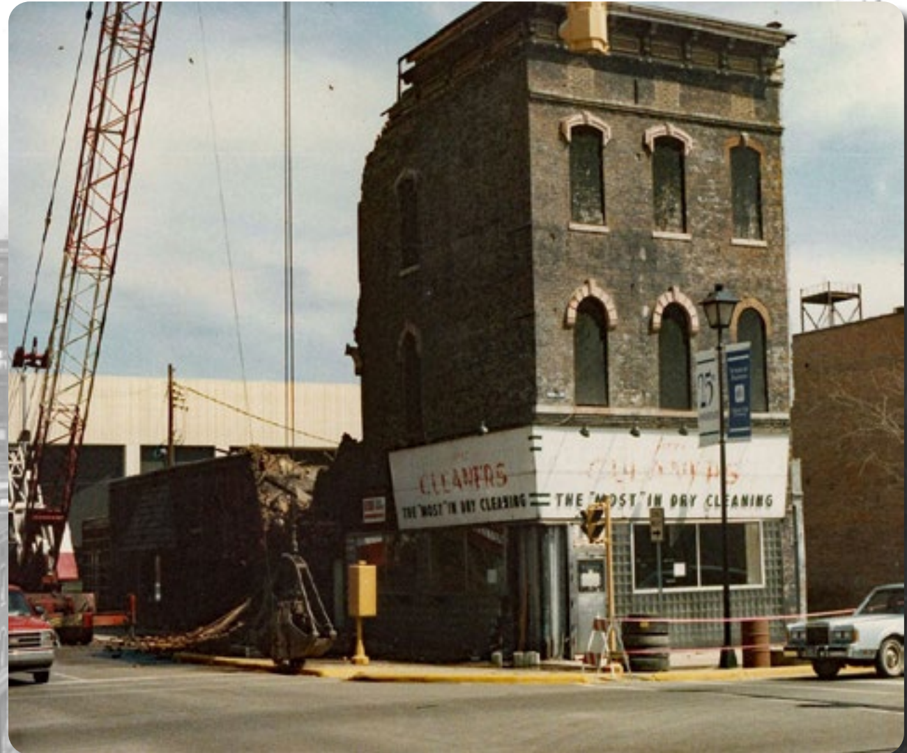
Demolition of the Washington Hall Circa 1990
