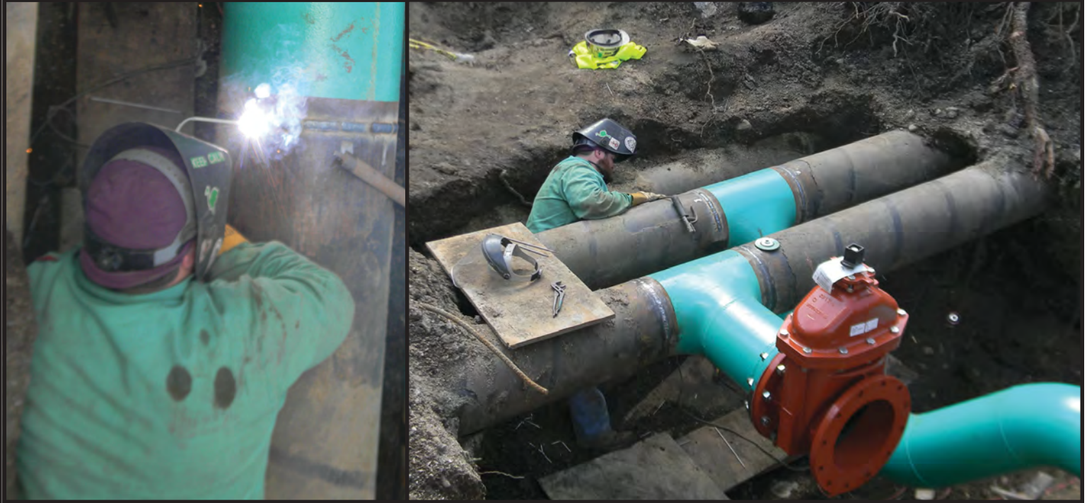
Corey Jackson working on the Underground Chilled Water Piping
